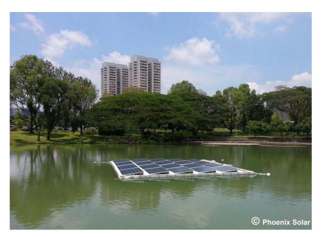
Caption: Phoenix Solar Pte Ltd has successfully connected to the grid the first floating photovoltaic (PV) system in Southeast Asia. The 5kWp system is a pilot project located in the Pond Gardens of Bishan Park.
